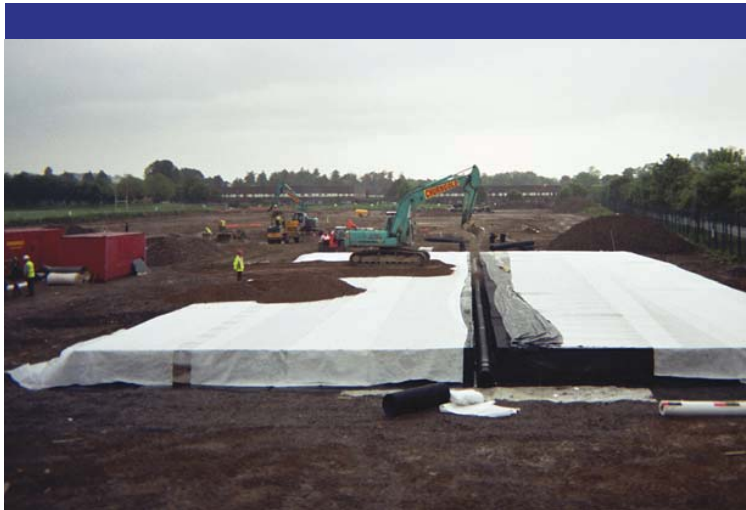
Typical stormwater attenuation system during installation.
